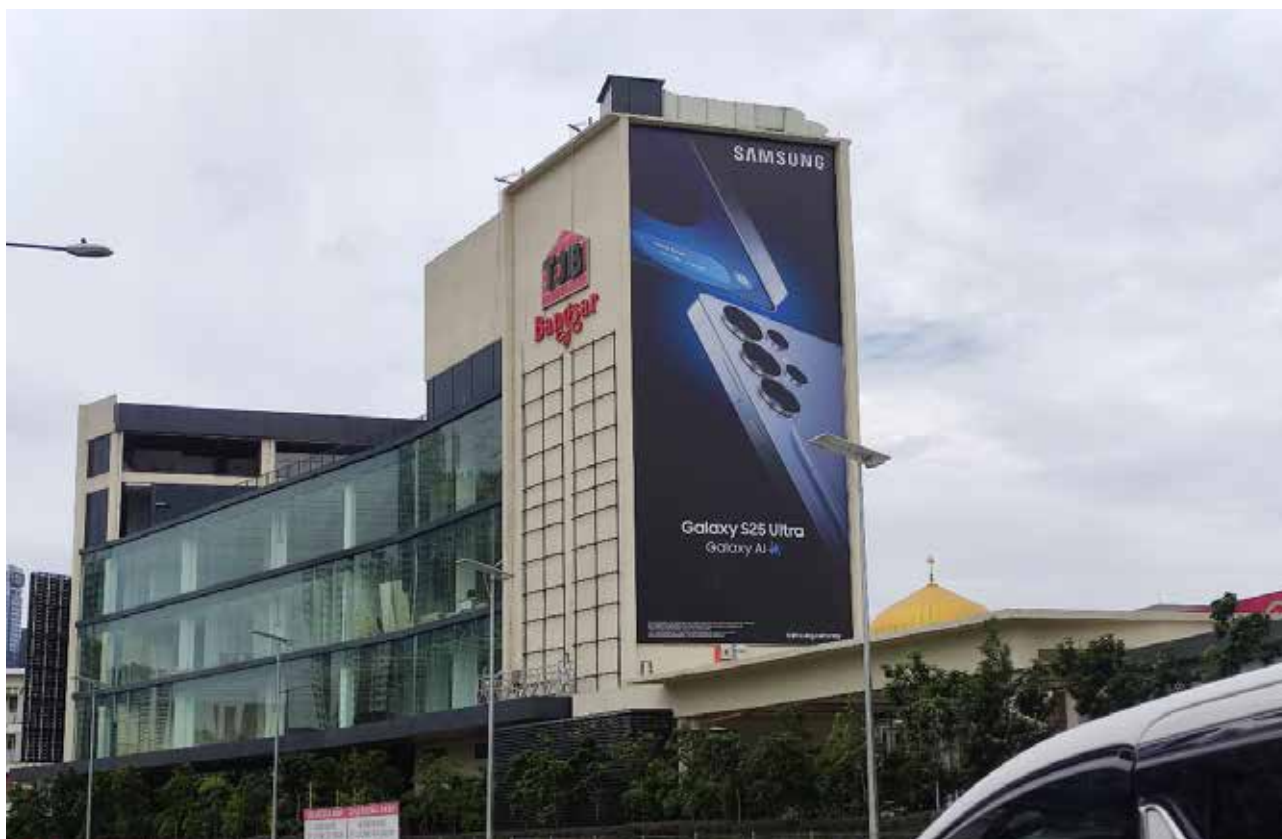
Static Wall Panel @ Bangsar
