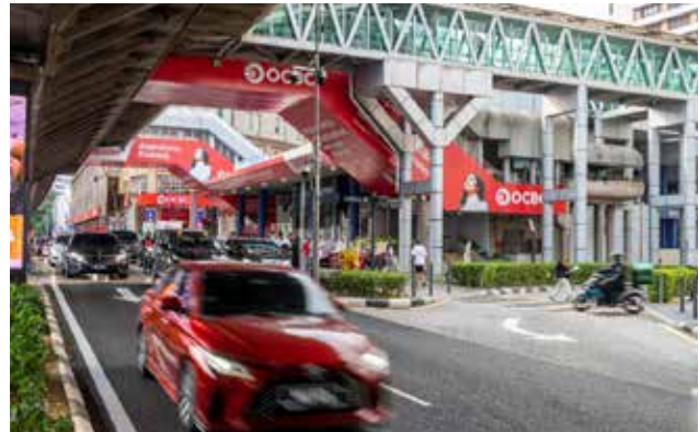
External Station Domination at LRT Masjid Jamek
