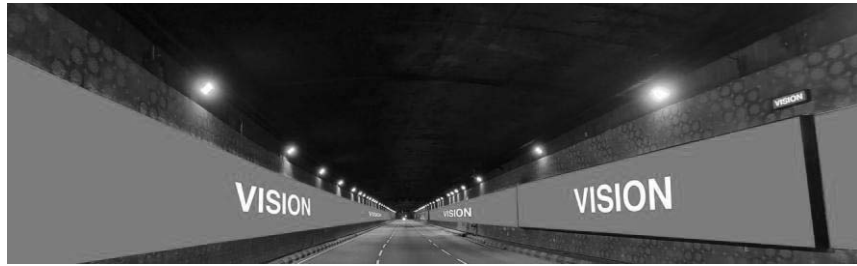
Tunnel wall panel
